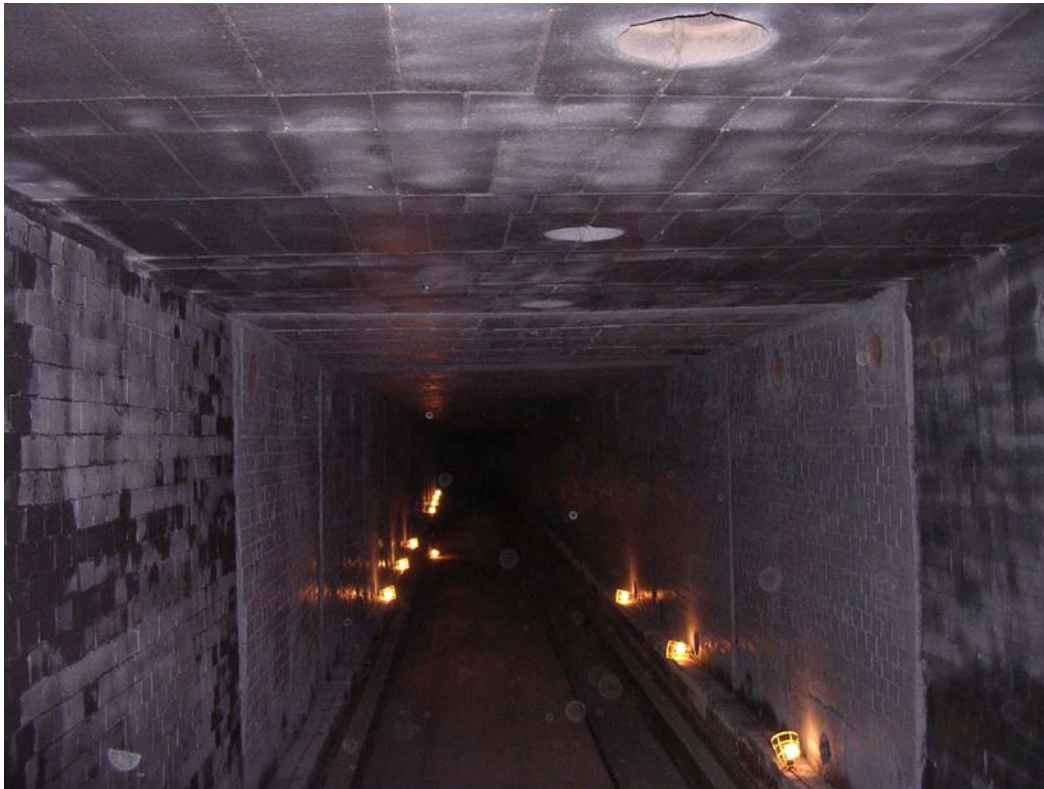
The kiln air-drying after completion of spraying Emisshield® ST-3
