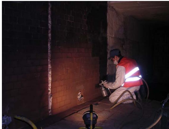
Spraying Emisshield® ST-3 on the firing zone walls
